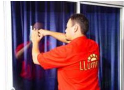
Wet the *adhesive only*, apply the precut film to dry glass, and aggressively squeegee application solution and air from beneath the film beginning from top center squeegeeing to one side or the other. Use ONE squeegee pass only, not multiple strokes over the same area. A Performax handle with Blue Maxx Squared blade must be used with uniform, very firm strokes. Using minimal overlaps, including the center, work any solution toward one side systematically from top to bottom.
