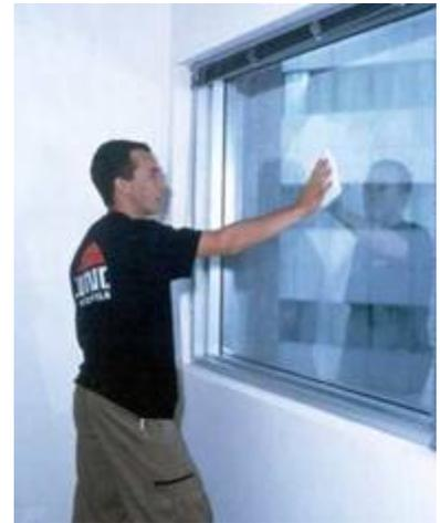
**REMINDER:** Never use a film installation squeegee as your cleaning squeegee, nor a soft bladed cleaning squeegee for an installation squeegee. Cleaning dirty glass will rapidly dull hard edges these blades. A hard, sharp edge must be maintained for installing film.
