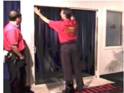
Two people working together can save several steps. In addition, their speed doesn't allow the application solution time to evaporate on either the window or the film during installation. This advantage reduces the need for frequent spraying, particularly on very hot days.
