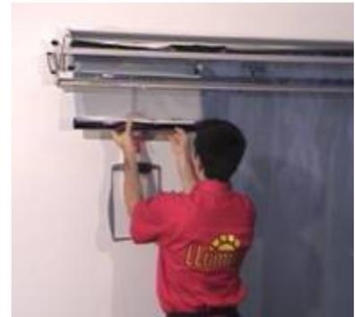
CPFilms recommends using two (2) six-foot stepladders for portable operations of the FilmHandler device. The massive weight of thick film rolls creates an unbalanced load on a single ladder and presents a safety hazard. Two ladders should be used for increased stability.
