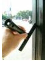
Spray the entire glass surface area with properly diluted X-100/Dirt-Off solution and use the 6" Triumph scraper to thoroughly scrape the entire window. Be careful
