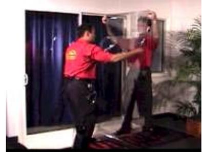
One person can clean the window while the other measures the window and prepares the film. One installer pulls the film from the box and holds it up for the desired length while the other cuts it.
