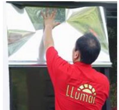
Uniformly spray the entire window surface, but avoid heavily spraying the top edge of the pane to prevent any contamination from flowing down from the border. Spray the exposed portion of the film with Film-On and grasp the film tube in preparation for lay up.
